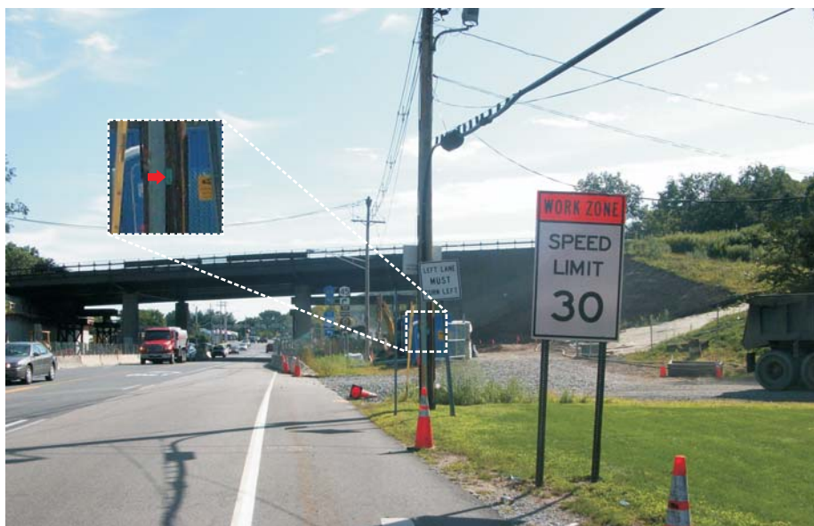
Figure 3.10-2: Photos of Long Trail Blazes Minisceongo Park
